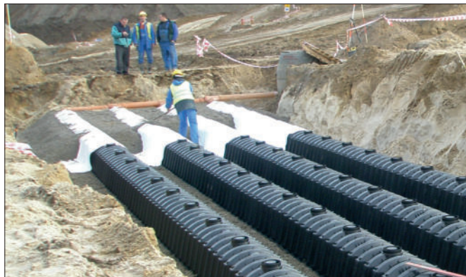
Figure 7 Installation of infiltration tunnels
